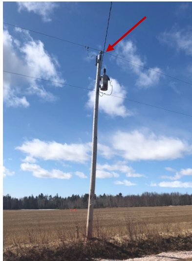
Penta-treated pole, old style insulator and old spacing.
