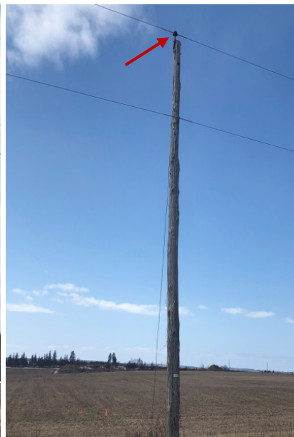
Cedar pole with old spacing and a small insulator.
