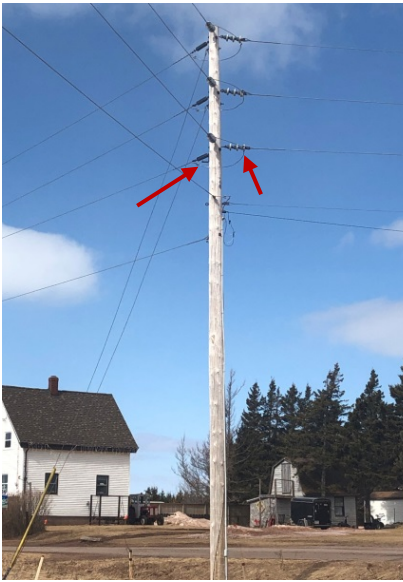
Penta-treated pole with two different dead-end insulators.
