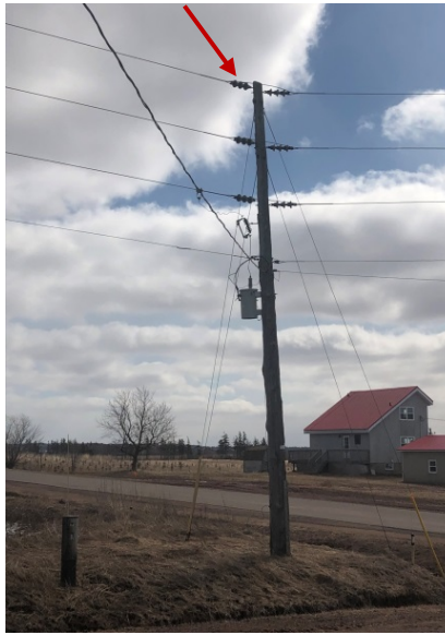
Cedar pole old dead insulators and old spacing.
