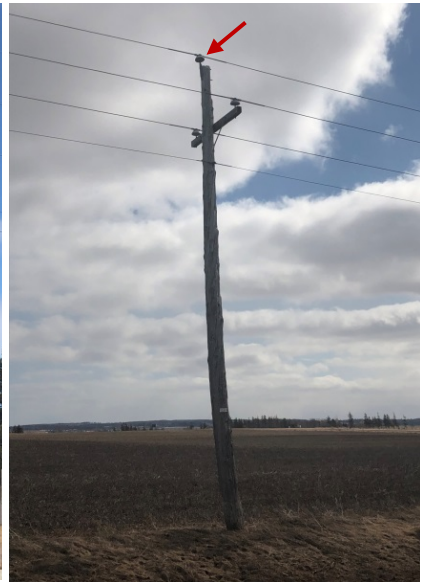
Cedar pole with old spacing and old style insulator.
