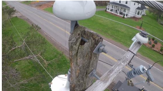
Figure 2-4: Poor condition pole top
