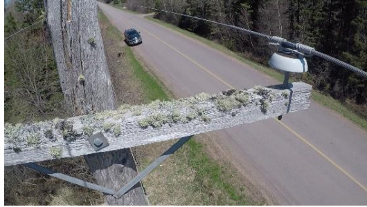
Figure 2-2: Deteriorated crossarm
