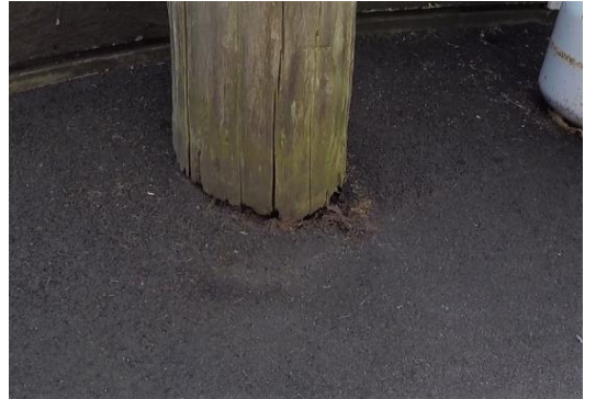
Figure 2-7: Severe decay in pavement
