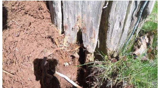
Figure 2-5: Severe below ground decay
