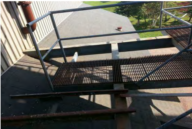
Roof view. Sloped Modified bitumen membrane.
