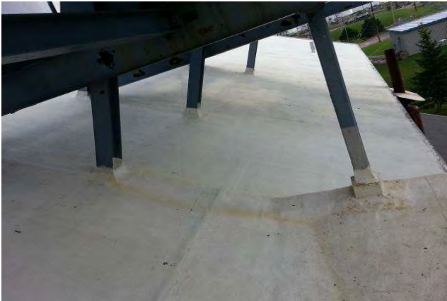
Roof view of North east side
