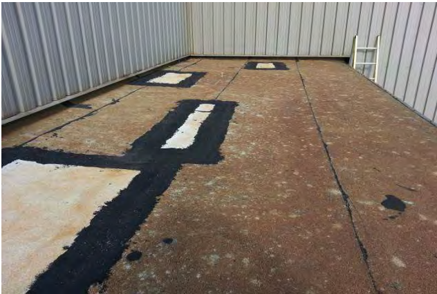
Roof view. Previous repairs are visible.
