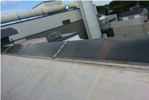
Skylights identified at roof ridge.
