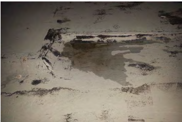
Aluminum pigment coating applied throughout roof surface. Roof Sleeper is coated.
