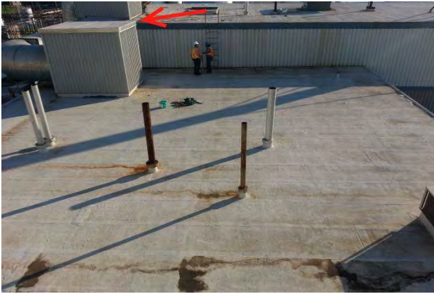
Penthouse roof area. No wet identified during thermal scan
