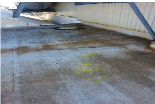
Daytime thermogram photo # 4
