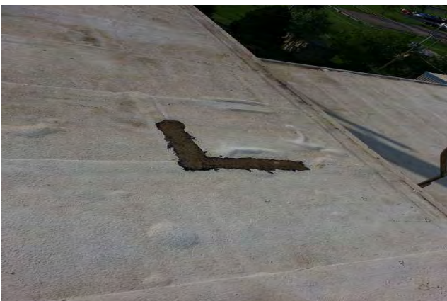
Previous roof repair is visible.
