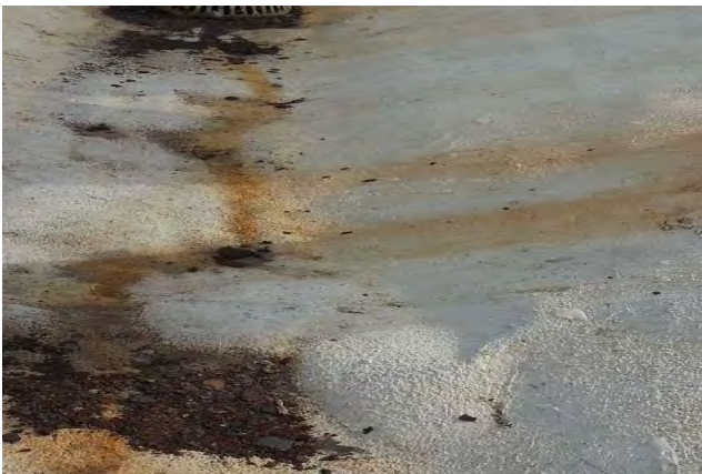
Debris visible at valley
