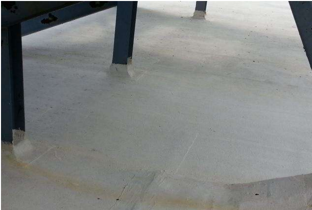
Roof view of North east side
