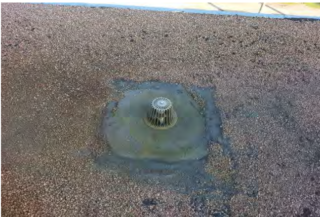
Drain flashing has been sealed with Modified Bitumen detail.
