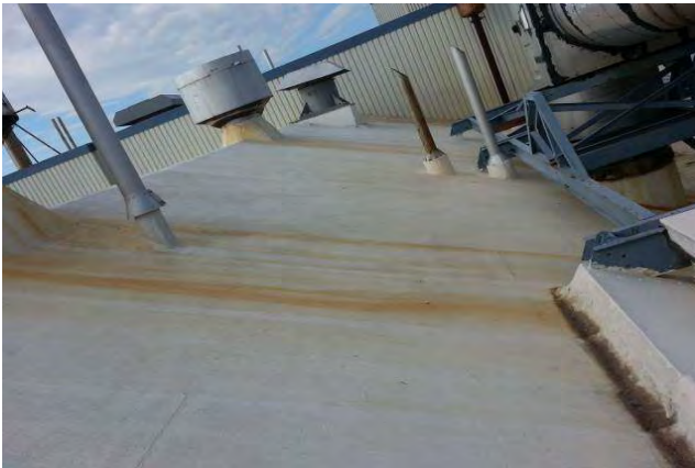
Roof view of south east side
