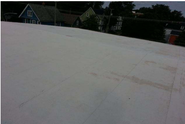
Roof view. Restorative fluid applied coating overtop Modified Bitumen roof surface.
