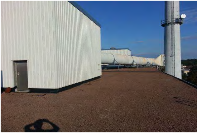
Roof View from North East corner
