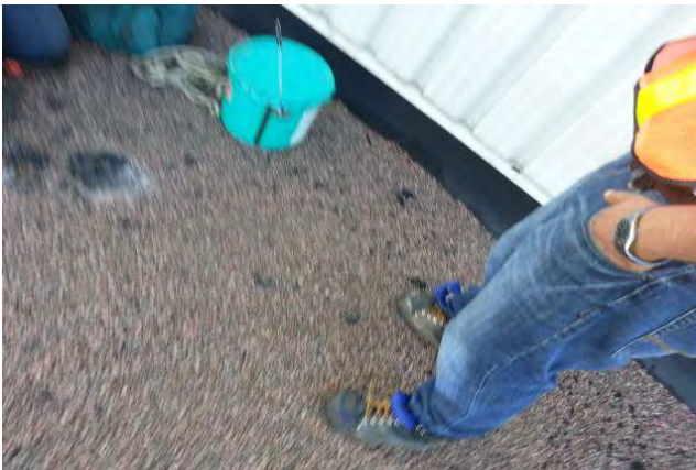
Verification cut performed to inspect for wet insulation. No wet identified.
