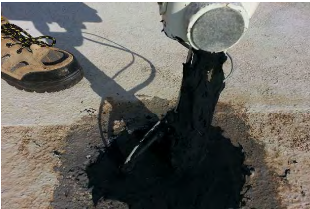
Monitoring camera mastic should be addressed.
