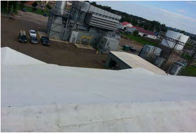
Roof view. No condition recorded. No access to roof area.
