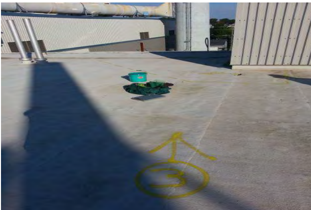
Daytime thermogram photo # 3.
