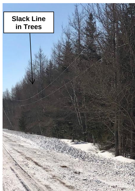
Primary line slack and laying in trees.
