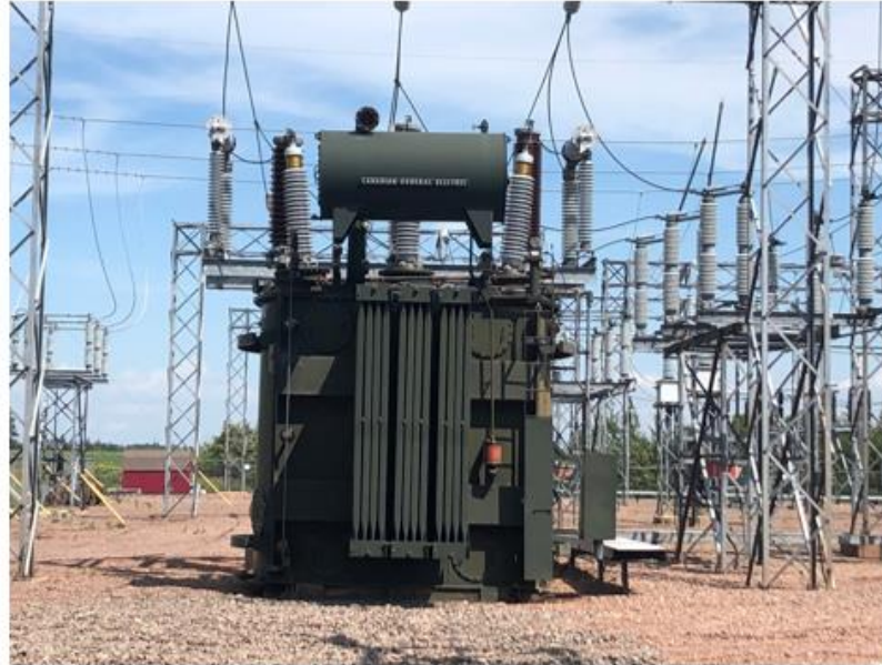
Bedeque 138 kV Reactor R1
