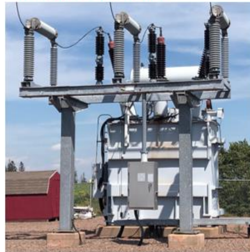
Bedeque 138 kV Reactor R1
