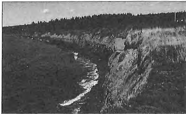
Figure 2. Example of cliff erosion at Cape Egmont
