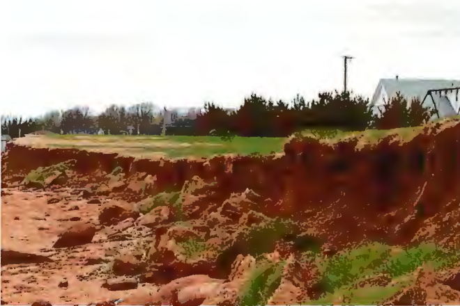
Figure 1. Example of bank erosion at Victoria's Provincial Park
