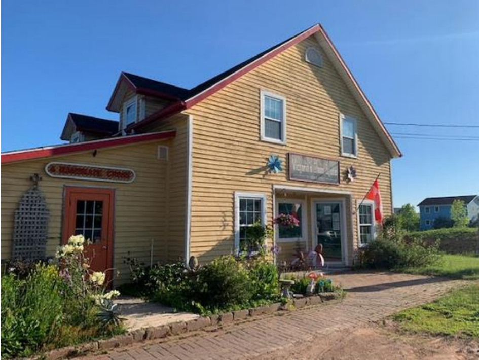
Plate 'C' - Existing building on the lot
